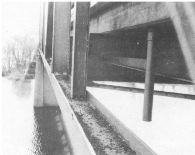
Figure 8-23. Lower chord of a riveted truss.
