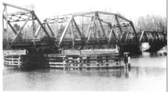
Figure 3-19. Timber bent fenders.
