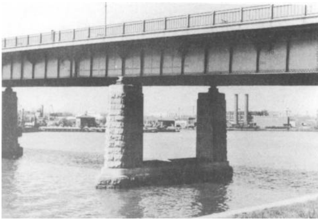
Figure 6-1. Nonload path redundant bridges.
