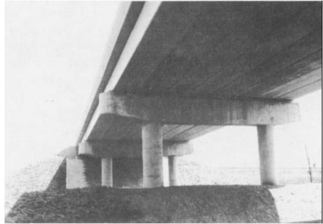
Figure 6-2. Load path redundant bridges.
