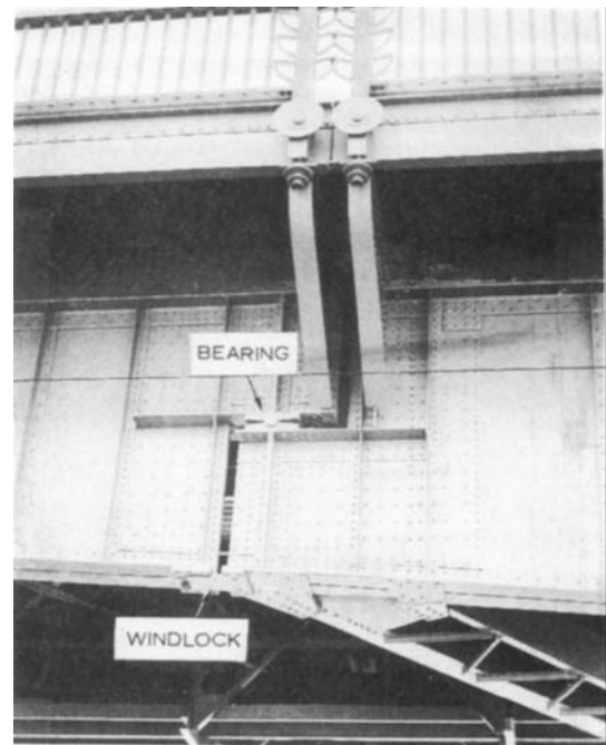
Figure 3-13. Bearing support for a suspended span.
