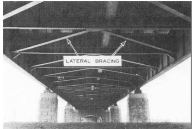
Figure 3-9. Bracing. (Sheet 2 of 2)
