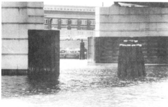
Figure 3-18. Timber pile cluster dolphins and timber fenders.
