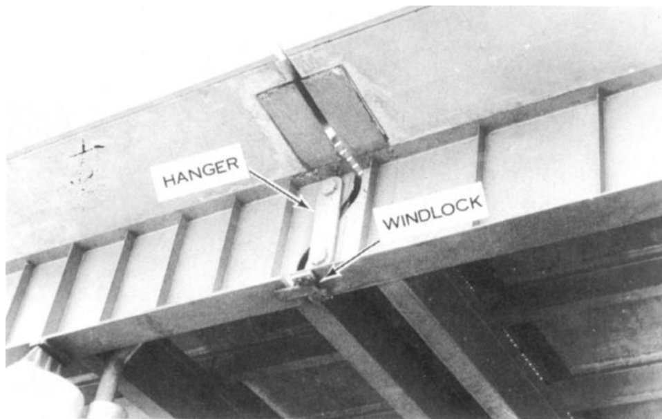
Figure 3-14. Pin and hanger connection.
